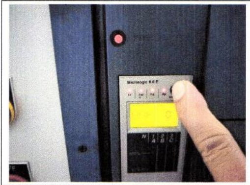
Picture 4: Electrical part replacement. (Battery Trip Unit Air circuit breaker)
