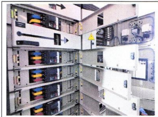
Picture 3: Main distribution board and preventive maintenance.
