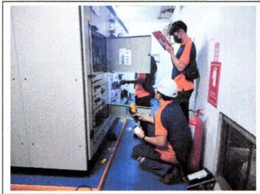
Picture 4: Main distribution board and preventive maintenance.
