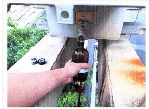
Picture 2: Oil type transformers and preventive maintenance.
